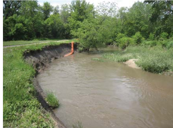
Severe streambank erosion, Duck Creek.
