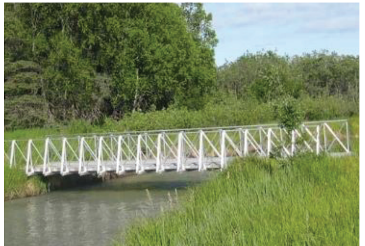
The bridges will be replaced with an aluminum framed version in 2019. This trail is used by hikers, bikers, and for horsebackriding.
