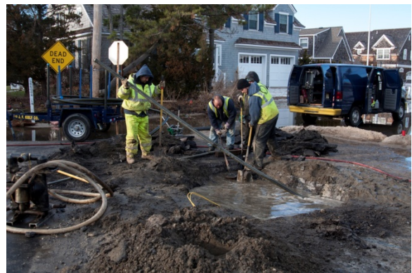
Photo: FEMA/Wendell Davis Jr.
