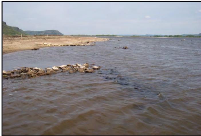
Photograph 4-14. J-Hook Vane in Pool 8
