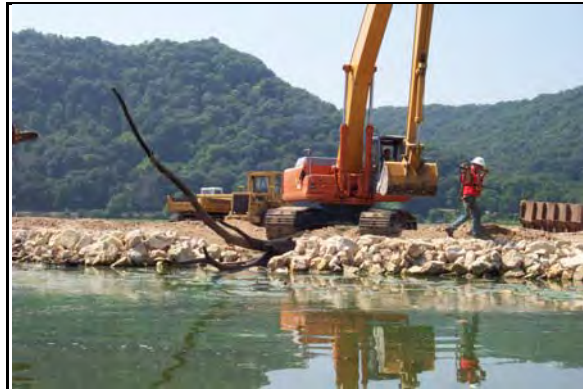
Photograph 9-15. Loading Structure Being Installed by the Contractor
