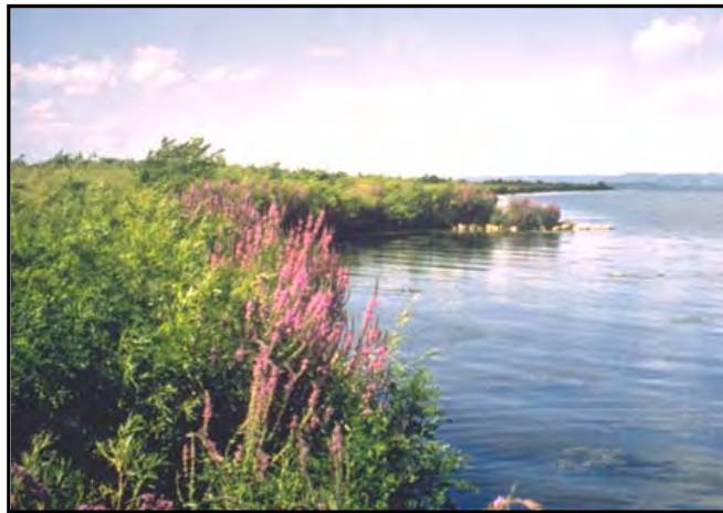
Photograph 4-12. Constructed Rock Groin in Pool 8 After a Few Years of Vegetation Growth)
