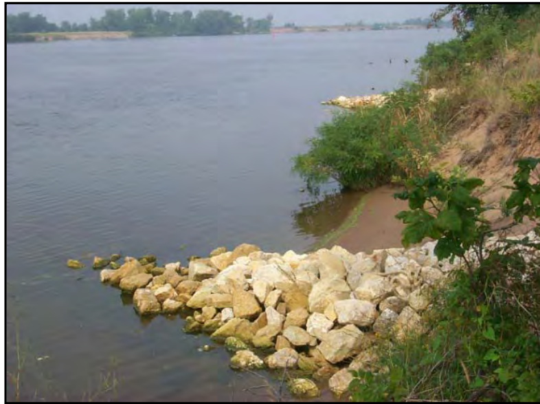
Photograph 4-13. Rock Vanes at Lost Island Chute, Pool 5
