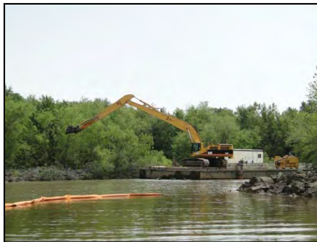
Photograph 6-15. Excavator Used To Dredge Back Channels
