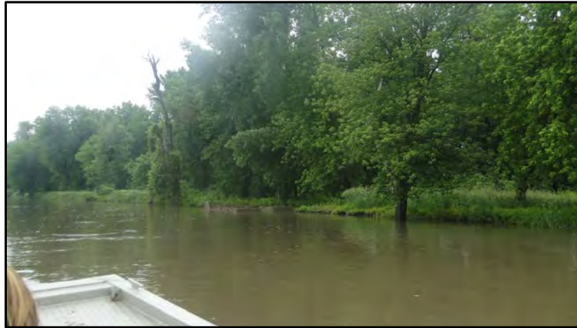
Photograph 4-6. Bankline Erosion at Huron Island, Pool 18 (note building foundation)
