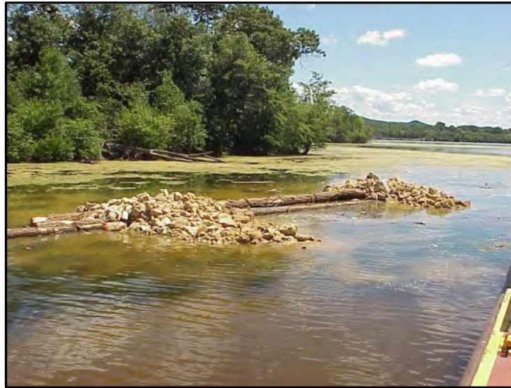
Photograph 4-17. Rock-log Structure in Place
