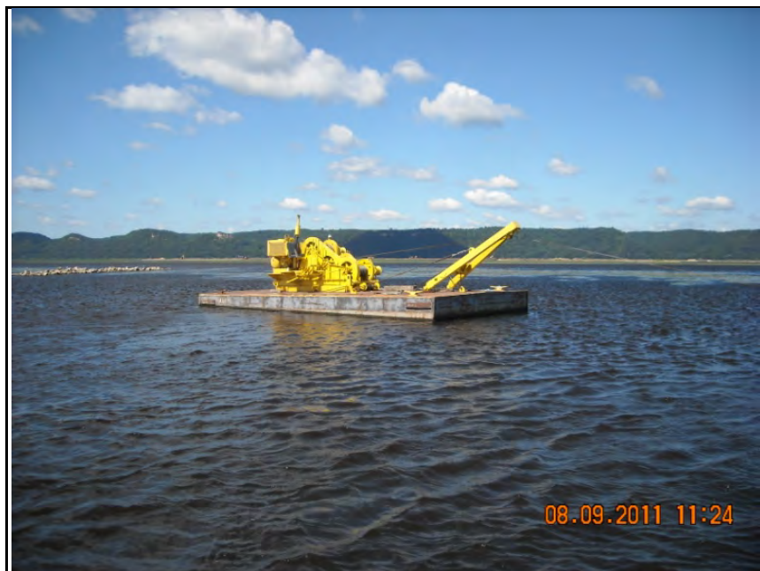
Photograph 9-F-3. Tugger Barge (used to hold pipeline in place)
