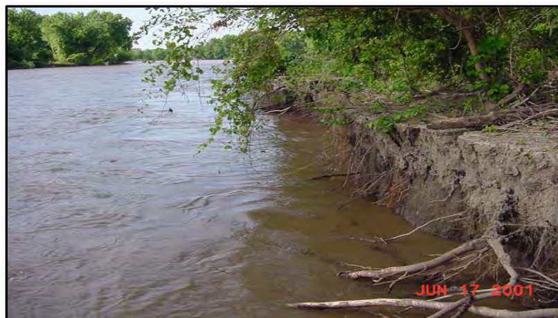
Photograph 4-7. Bankline Erosion on Long Island Division, Pool 20
