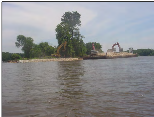
Photograph 4-9. Placement of Rock Revetment at Long Island
