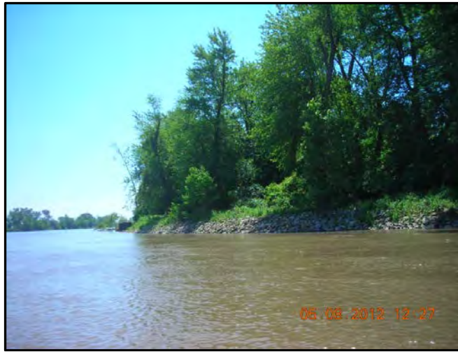
Photograph 4-10. Area of Rock Placement at Long Island 8 Years Post Construction
