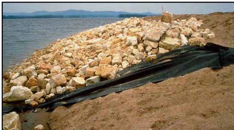
Photograph 4-2. Riprap and Geotextile Filter Placed on Sand (Lake Onalaska)
