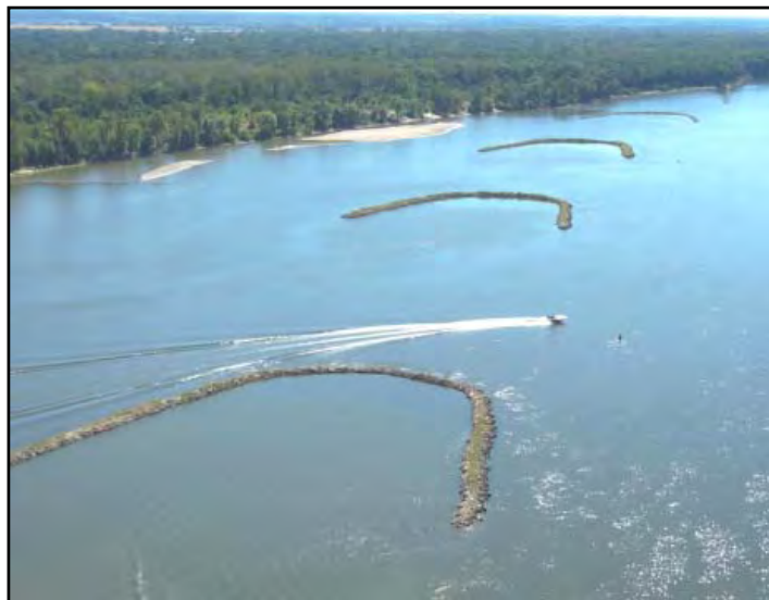
Photograph 7-8. A Series of Chevrons Aligned To Split Flow Between the Main Channel and a Side Channel, While Protecting the Existing Shoreline
