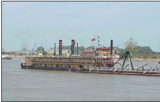
Photograph 7-19. Dredge Using Hydraulic Pipeline
