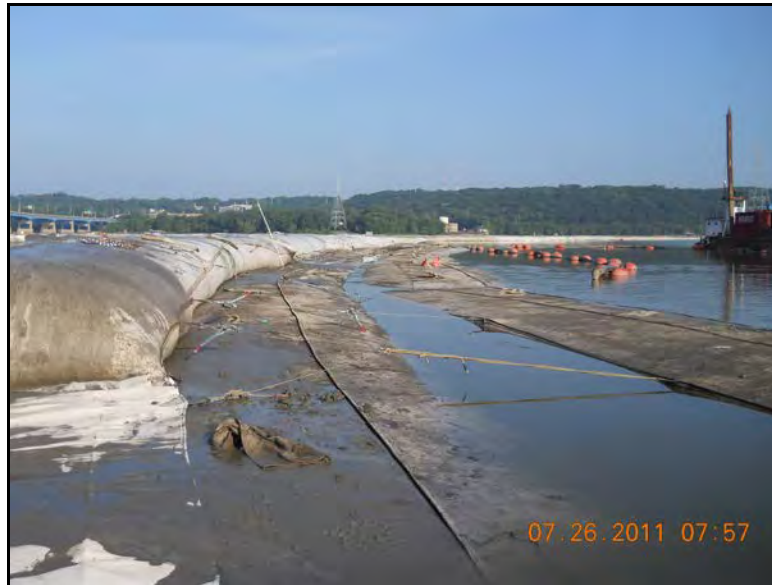
Photograph 6-5. High Solids Geotextile Containers Placement Peoria, IL
