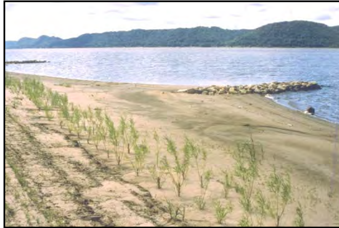
Photograph 4-11. Newly Constructed Rock Groin in Pool 8
