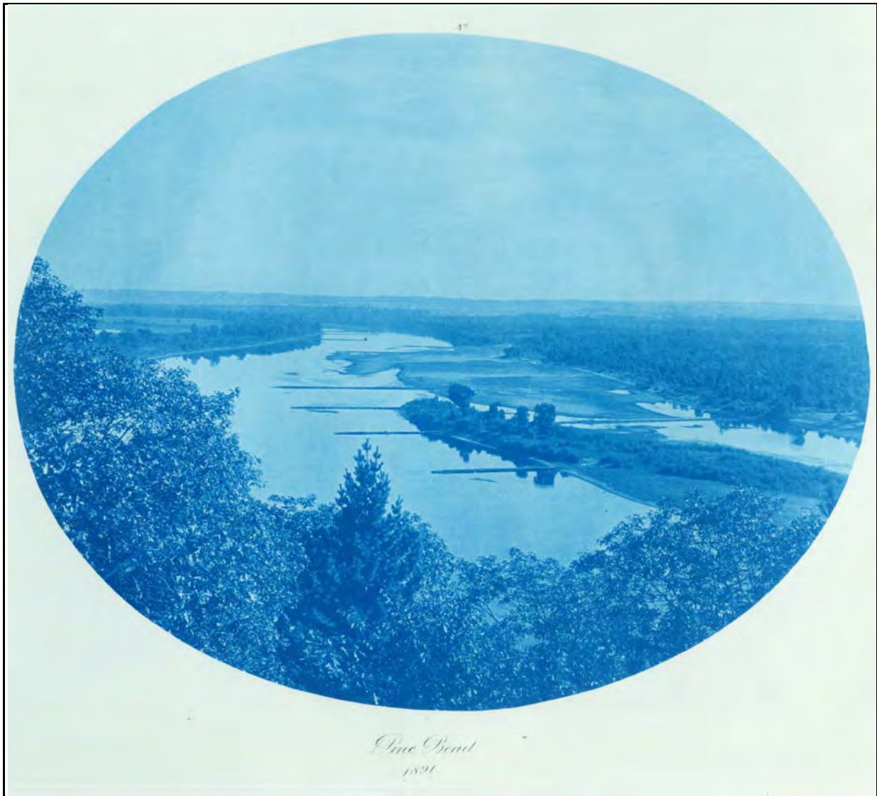
Photograph 9-1. Wing Dams at Pine Bend by Henry Bosse The navigation channel is to the left of the main channel Sediment accumulation in the “field” of wing dams can be seen near the center of the photograph.
