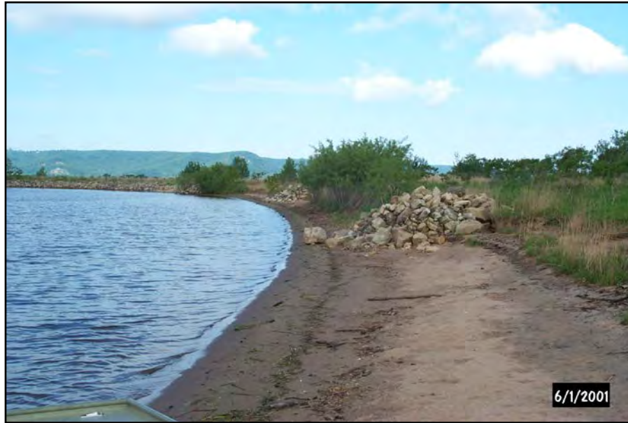
Photograph 9-C-1. Ice Damage to Groins Constructed at Lake Onaska, Pool 7
