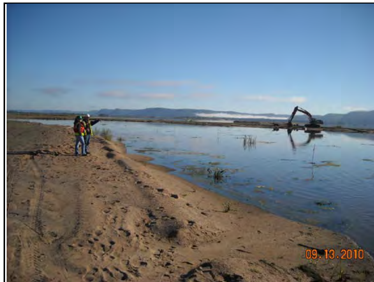
Photograph 9-F-1. C4 Mudflat – Stage 3A (Emergent Wetland Under Construction)
