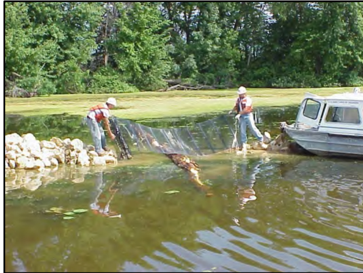
Photograph 4-16. Installation of a Rock log Structure
