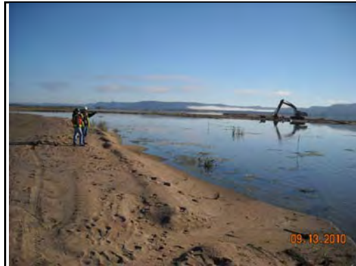
Photograph 9-14. Pool 8, Phase III, Island C4 Mudflat During Construction
