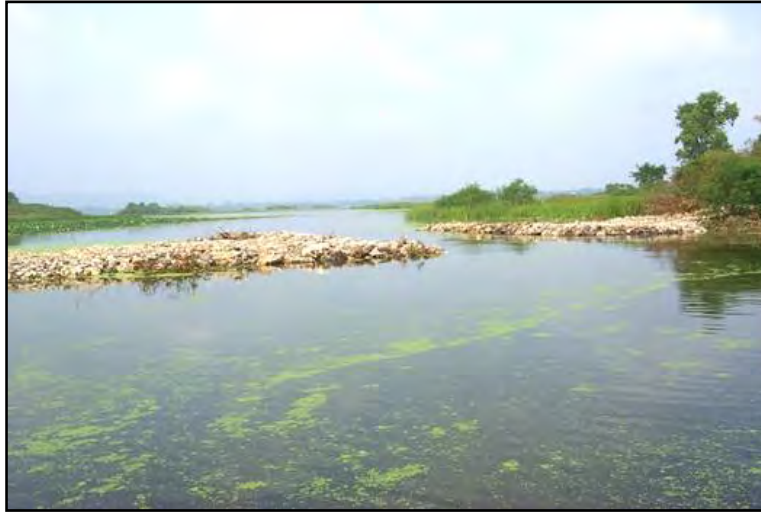
Photograph 7-1. Partial Closure Structure at the Weaver Bottoms Secondary Channel, Pool 5 (Jon Hendrickson, MVP 2005)
