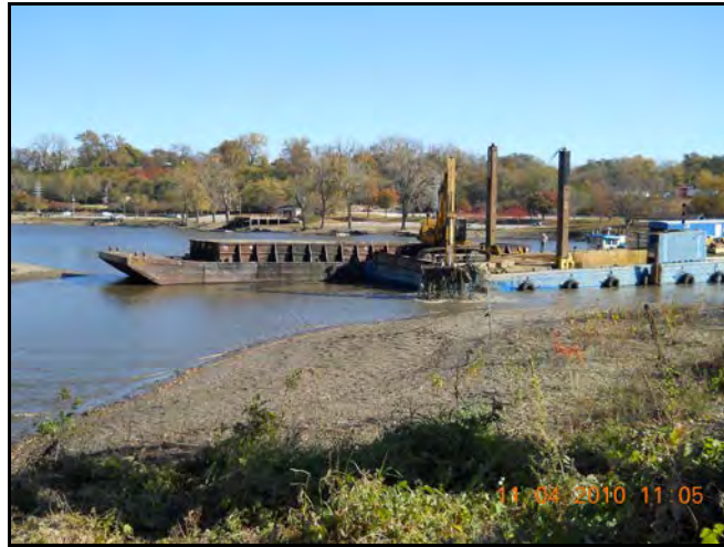
Photograph 6-2. Mechanical Dredging in Quincy Bay Harbor Quincy, IL
