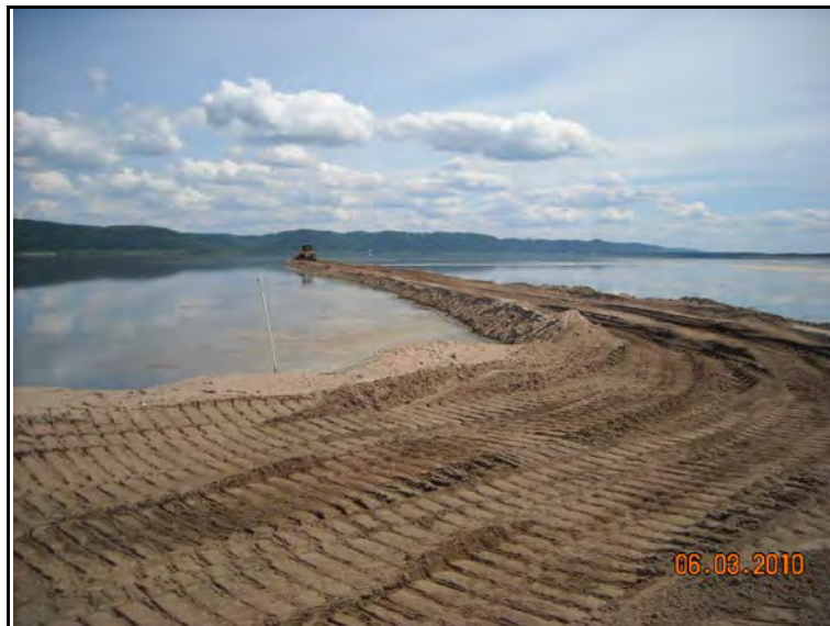
Photograph 9-F-5. Construction of a Permit Approved Access Road, Stage 3A Project
