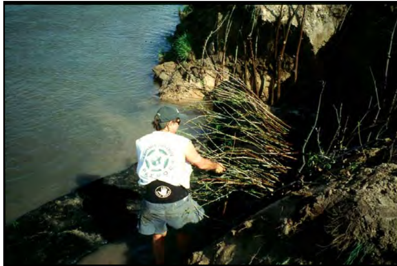
Photograph 7-22. Bioengineering Using Willow
