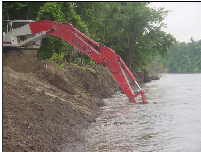
Photograph 4-8. Long Island Bankline Prior to Rock Placement
