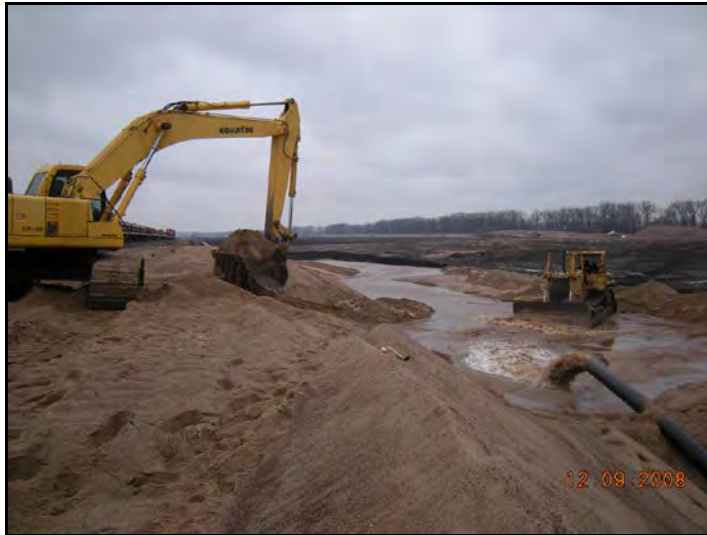
Photograph 6-3. Hydraulic Dredging Material Discharge at La Grange, MO
