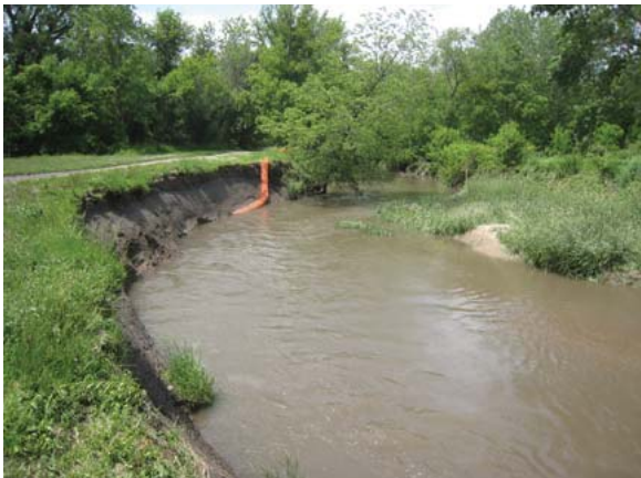
DW 12: severe erosion within Junge Park threatens the recreational trail.
