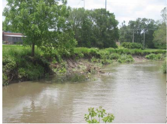
DW 11: severe bank erosion and slumping near Brady Street.
