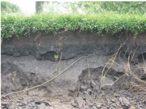
DW 12: turf grass does little to stabilize stream banks.
