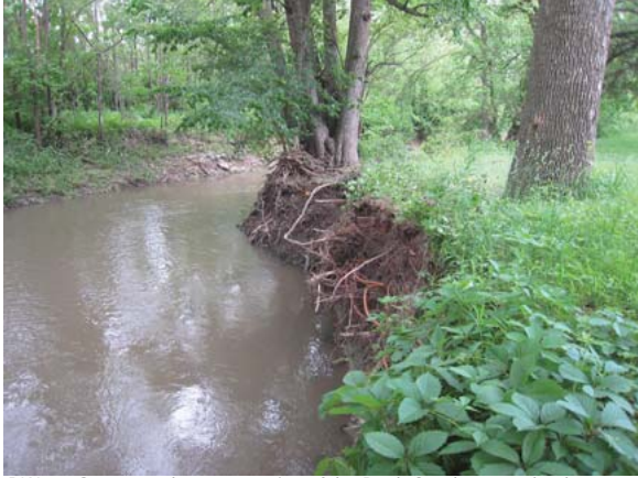
DW 10: Severe and recent erosion of the Duck Creek stream banks.
