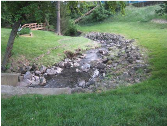
RR2.16: rock armoring is often used to stabilize eroding streambanks.
