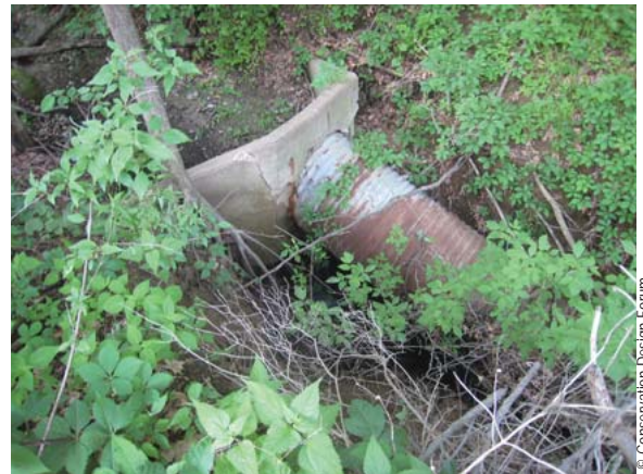
RR3.3: erosion can expose and damage stormwater infrastructure.
