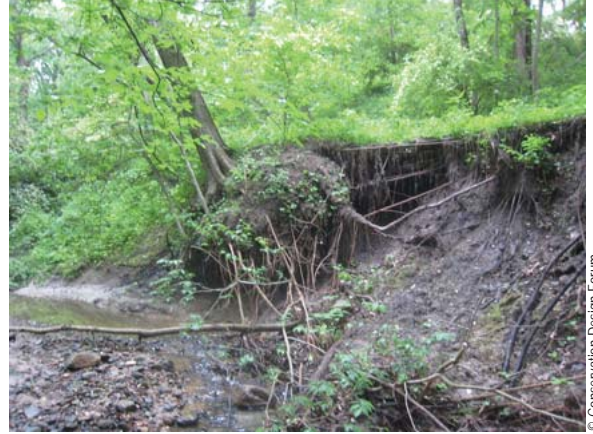
RR6.3: streambank erosion
