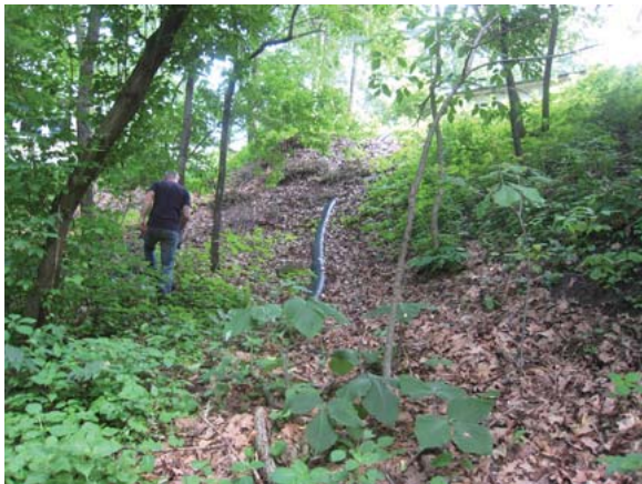
RR5.11: yard waste and residential drain pipes cause ravine and stream degradation but are easily addressed.
