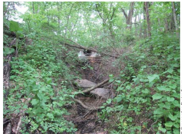
RR3.5: erosion below a stormsewer outfall.
