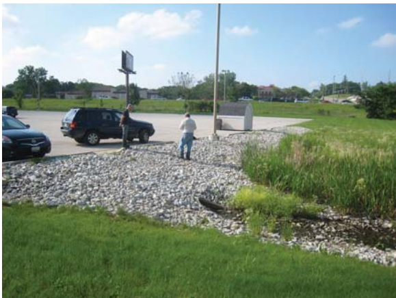
RR3.9: this rock and wetland facility helps cleanse and retain stormwater runoff from the adjacent parking lot.
