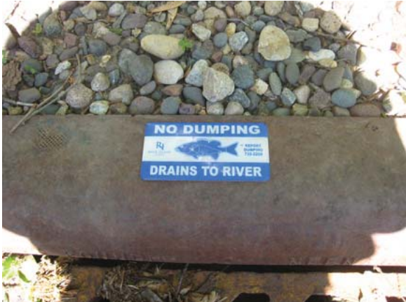
RR3.6: stormdrain labeling can help educate residents and landowners about the impacts of their actions.
