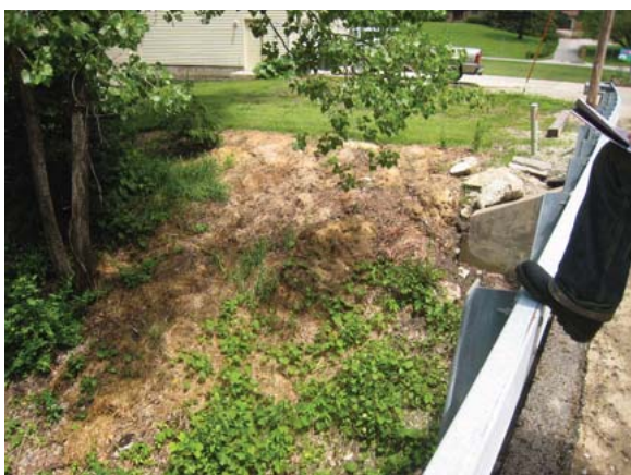
RR2.4: dumping of yard waste along ravines.
