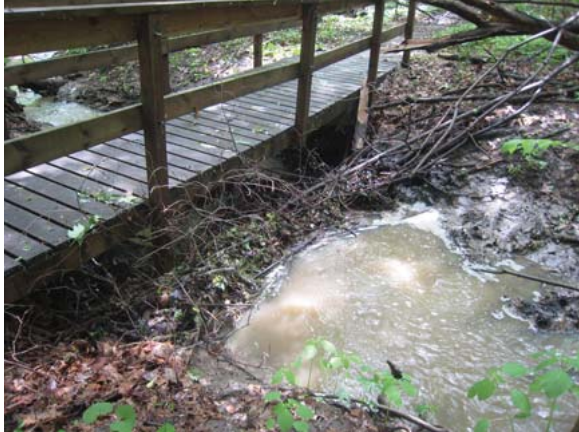
RR2.1: debris jams can worsen erosion as water flows around them.
