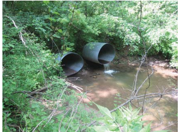
RR4.3: twin stormwater outfalls.
