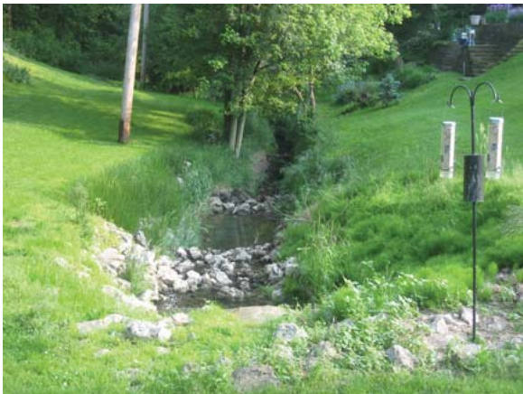
RR3.7: a streambank stabilization project.
