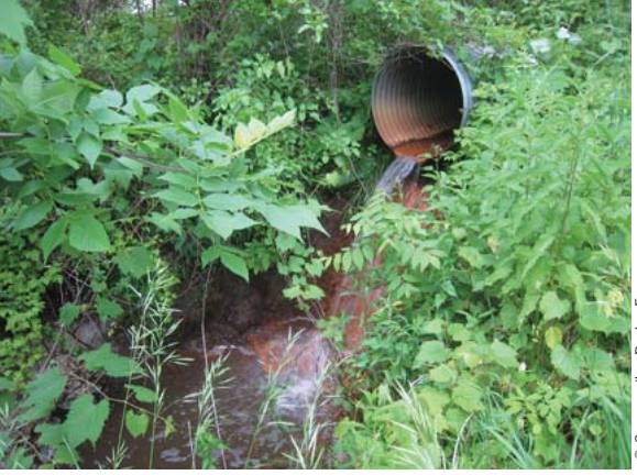
RR10.3: this stormwater discharge is creating an eroded plunge pool.
