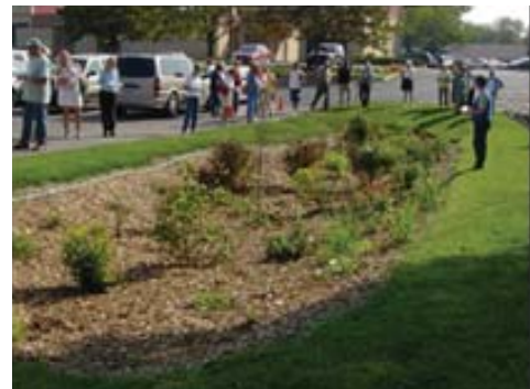
rain garden designed to filter and infiltrate parking lot runoff (Rock Island, IL)
