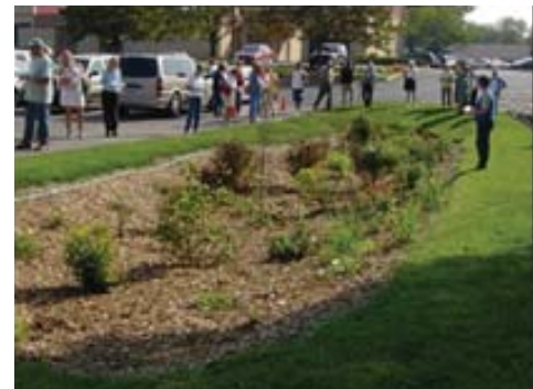
rain garden designed to filter and infiltrate parking lot runoff (Rock Island, IL)
