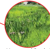
Vegetated Swale/ Rain Garden
