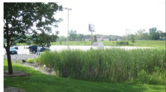
this swale receives runoff from the parking lot in the background (Rock Island, IL)
