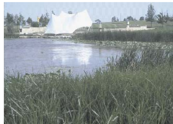
a well designed naturalized wet detention pond provides open space and passive recreation opportunities
