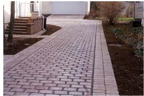
Porous Pavement (Elmhurst, IL)
