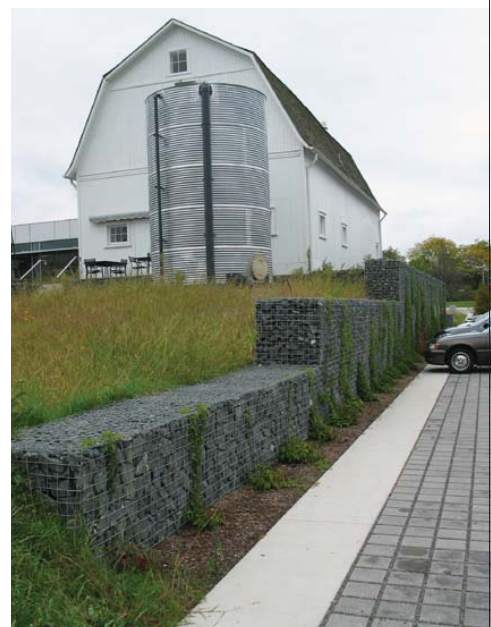
a cistern system collects rainwater from Kresge Foundation Headquarters (Troy, MI) (Photo: Conservation Design Forum)
