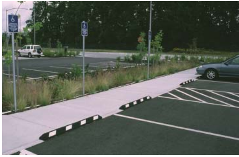
Bioswales along streets (Portland, OR)
